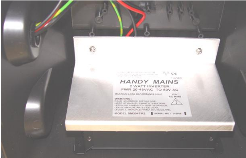
Figure 6 - Installation of Inverter Bracket
