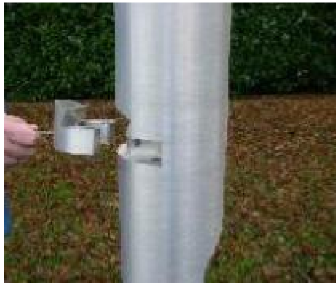
Figure 9 – Hinged Pole Wedge Removal
