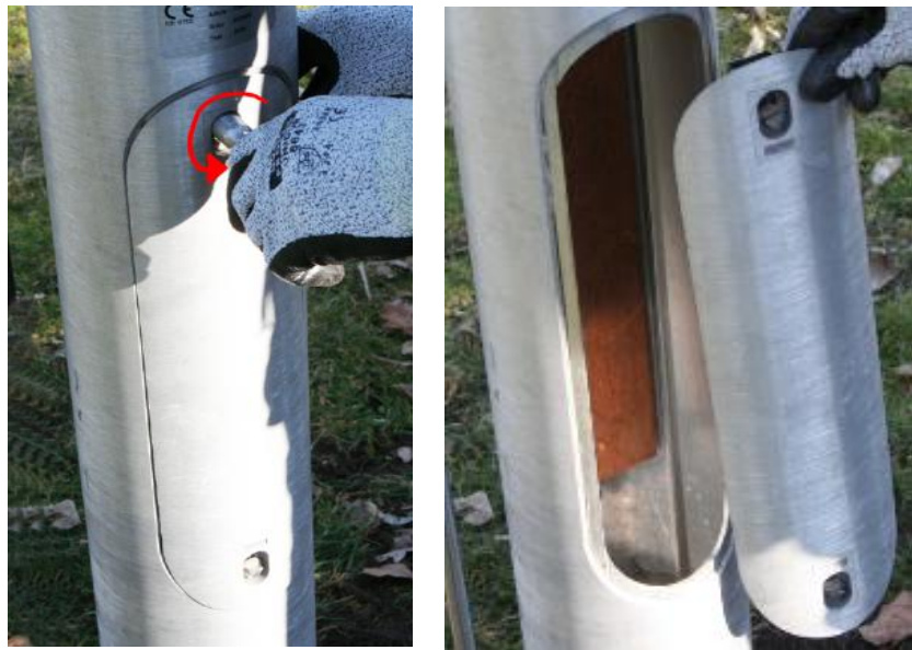
Figure 3 - Sapa Hinged Pole Door Removal
