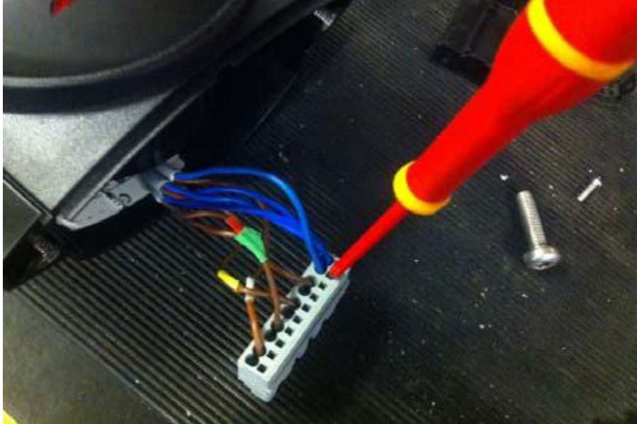
Figure 9 – Release return core for Regulatory Sign
