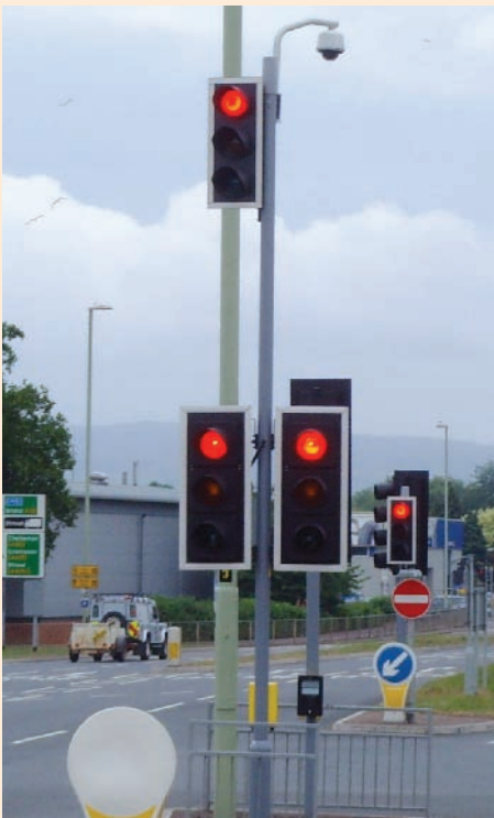
Telscan installation in Gloucester
