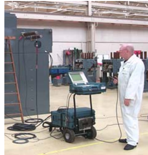
Pf Testing of Capacitor Bushings
